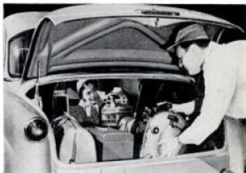
HUDSON Jet has a removable rear seat. With it out, trunk divider wall drops to make huge loading area
